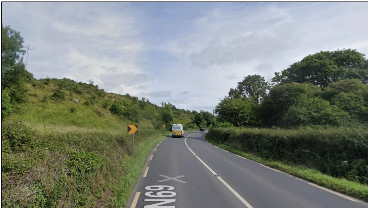
Figure 4-5: Photograph 2 of Pinch Point 2
