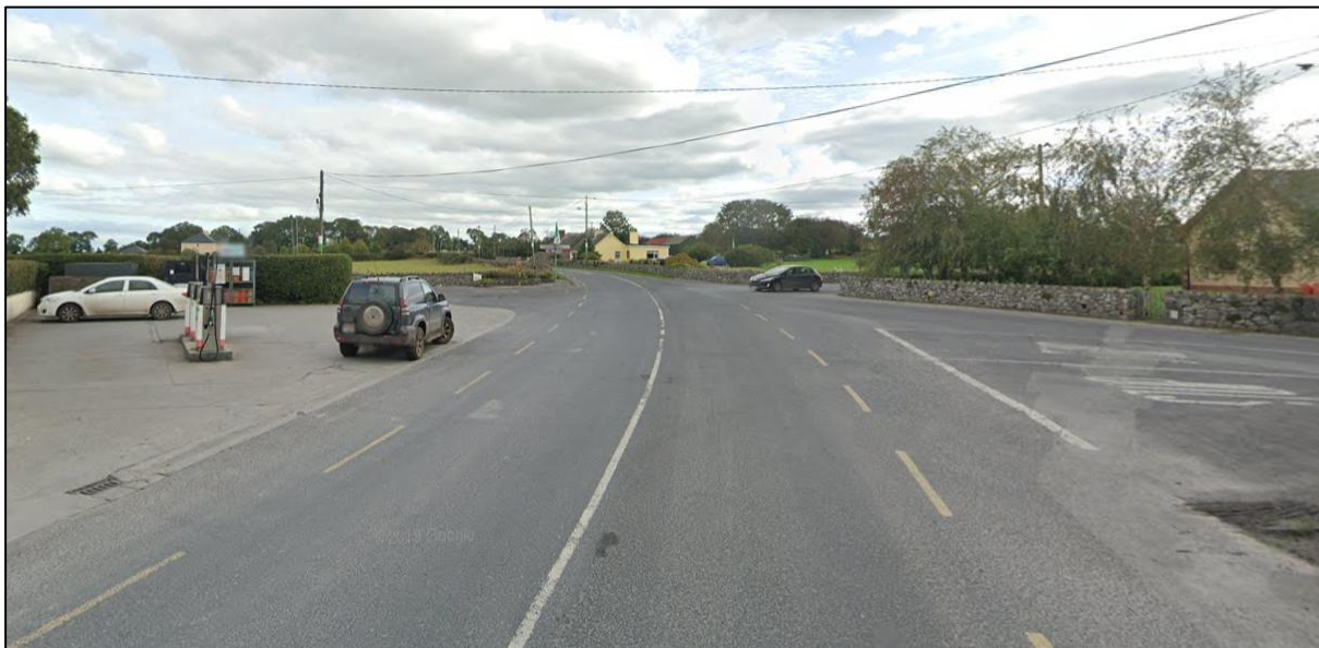
Figure 4-15: Photograph of Pinch Point 7
